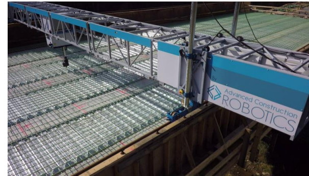
Figur: Rebar-Tying Robot. TyBot LLC sier: «No pre-mapping, programming or calibration required. TyBot self-locates, self-positions and self-ties the rebar intersections (Kilde: www.tybotllc.com )
