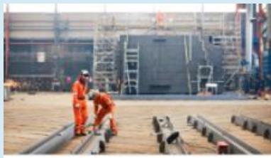
Construction and Commissioning
