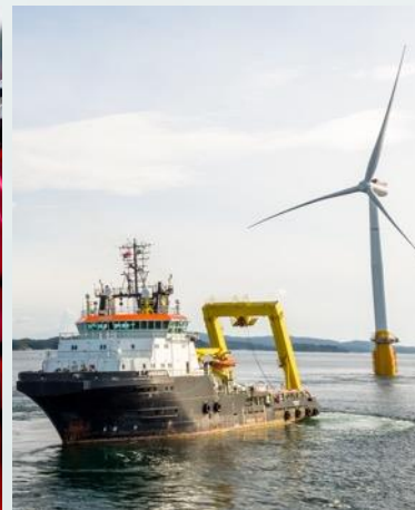
Marine operations & maintenance
